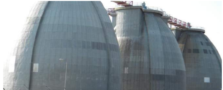
Glina wastewater treatment plant
