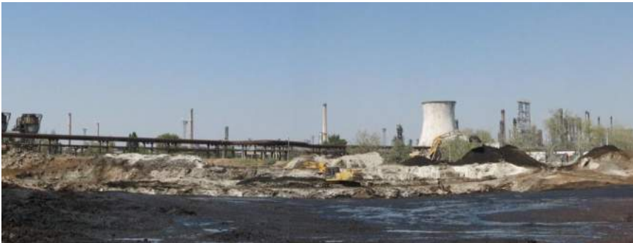
Petrobrazi refinery internal lagoons cleanup Remediation
