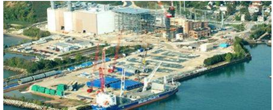
Port Washington Generating Station, Wisconsin, USA
