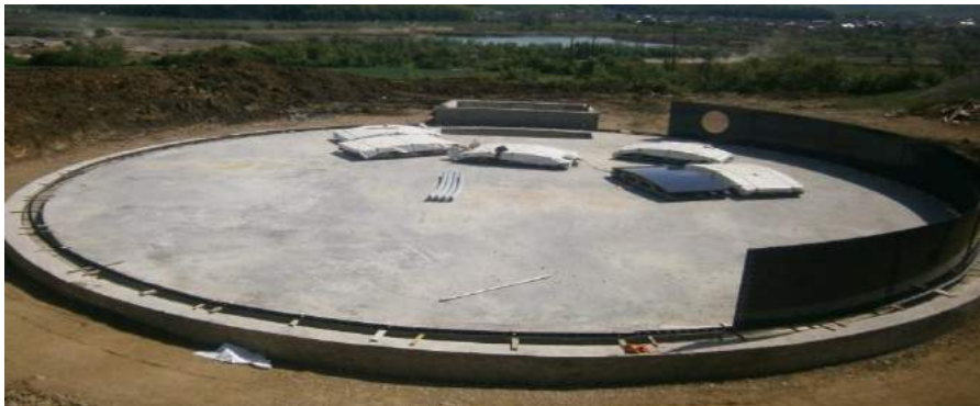
Extension and renovation of water and wastewater infrastructure in Hunedoara County
