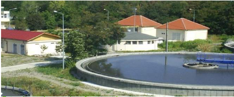
Extension and renovation of water and wastewater infrastructure in Neamt County
