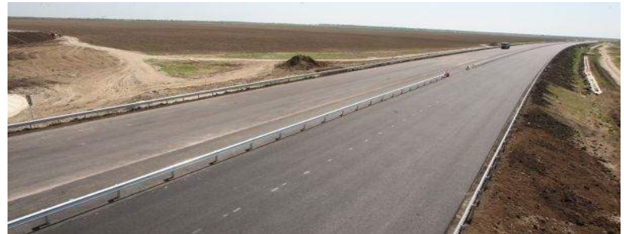
DN56 and DN56A – design and construction supervision
