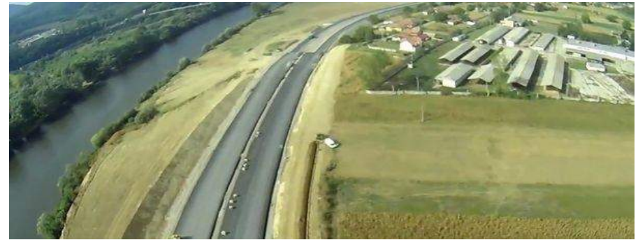
Deva-Orăștie – construction supervision
