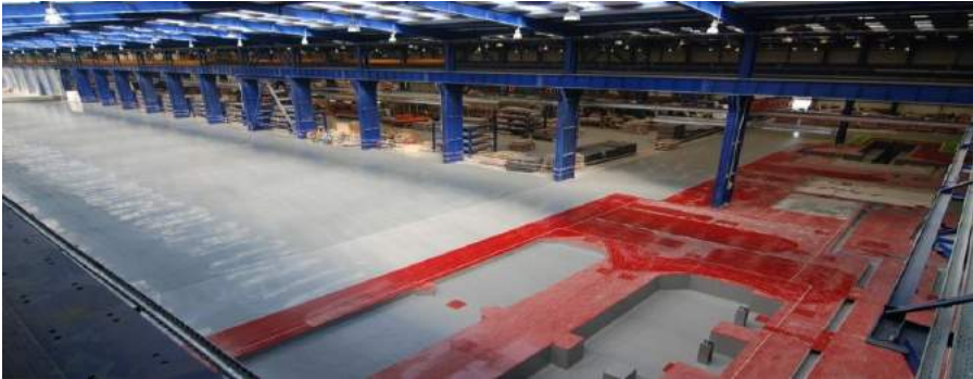
Bamesa steel services center, Arges County
