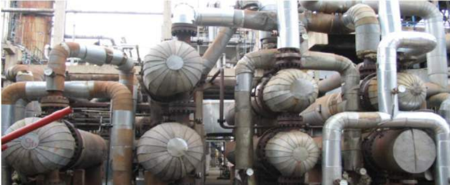
Brazi refinery turnaround, Romania – management and project controls
