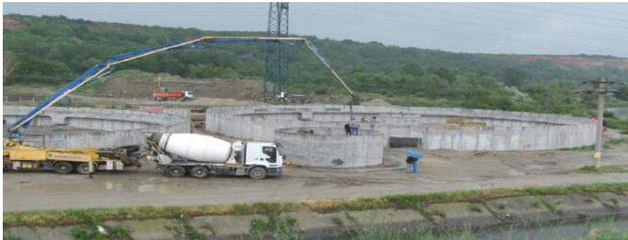
Extension and renovation of water and wastewater infrastructure in Olt County
