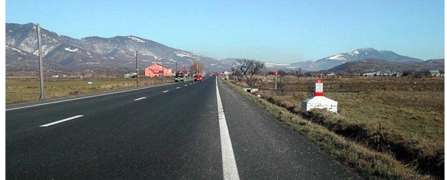
DN1C and DN17 – design and construction supervision
