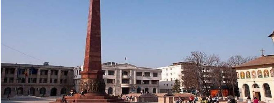
Focsani City Center renovation
