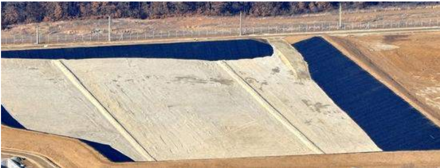
JTicleni bio-treatment plant and landfill, Gorj County Construction
