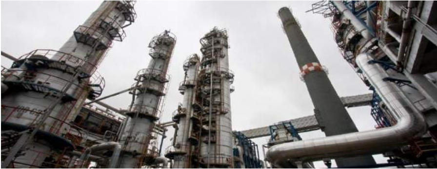
Petromidia Gasoil Drying Unit, Romania
