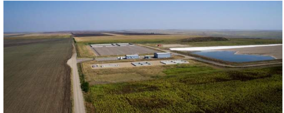
Independenta bio-treatment plant, Galati County Construction
