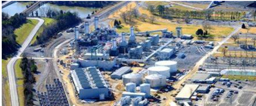
John Sevier CC Plant, USA – award winning project, Top Plant of 2012
