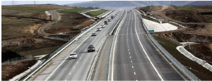
Lugoj-Deva section 4 – construction supervision
