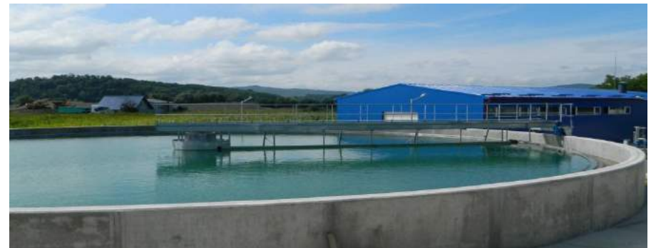
Extension and renovation of water and wastewater infrastructure in Bistrita-Nasaud County
