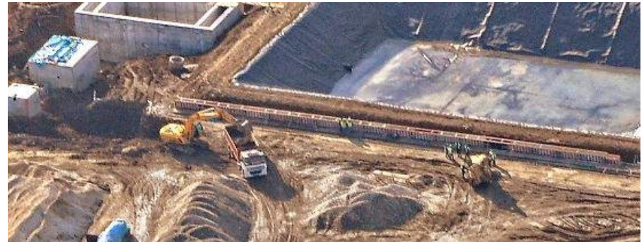
Barasti bio-treatment plant, Olt County Construction
