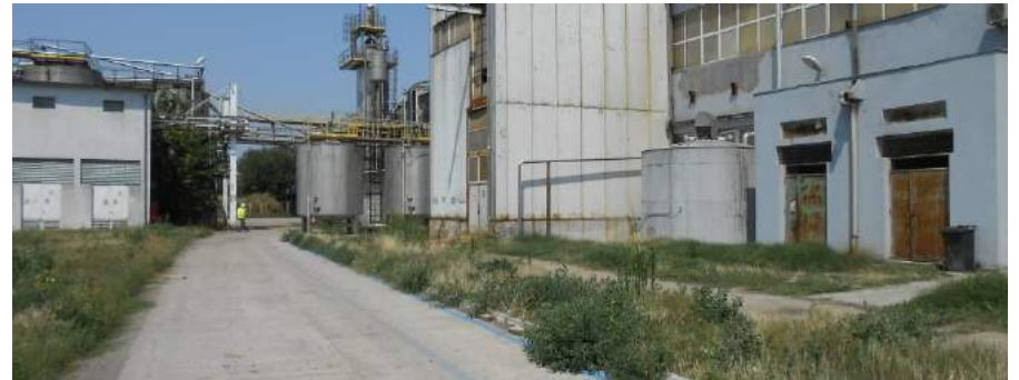
Food industry plant decommissioning
