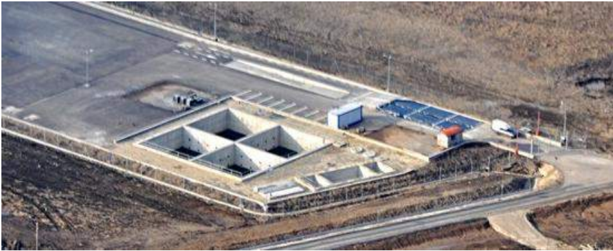
Videle bio-treatment plant, Teleorman County Construction
