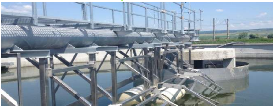
Extension and renovation of water and wastewater infrastructure in Brasov County
