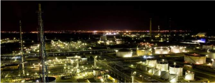
Petromidia Kerosene Hydro-treating Revamp, Romania
