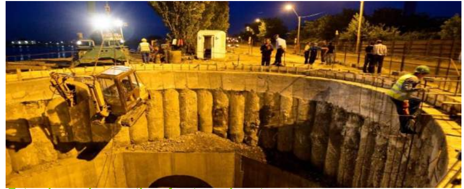
Extension and renovation of water and wastewater infrastructure in Arges County
