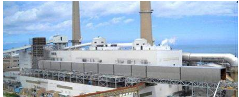
South Oak Creek Power Plant, Wisconsin, USA
