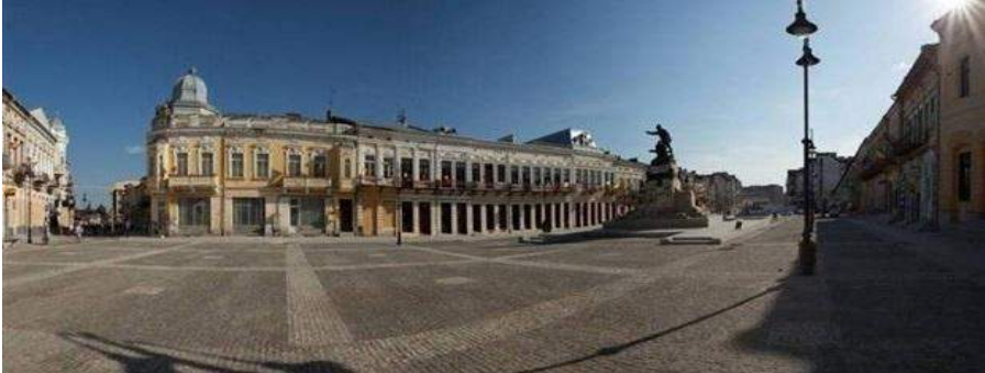
Botosani City Center renovation
